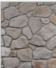
laid with mortar color "Ash Gray"
