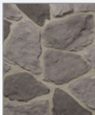
laid with mortar color "Ash Gray"
