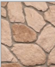
laid with mortar color "Ash Gray"
