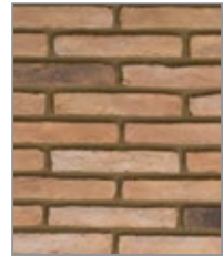
laid with mortar color "Mocca Brown"
