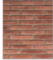
laid with mortar color "Ash Gray"
