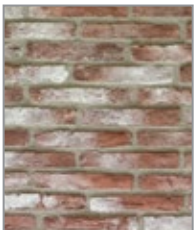
laid with mortar color "Ash Gray"
