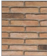
laid with mortar color "Ash Gray"
