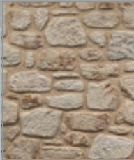
laid with mortar color "Coral Sand"
