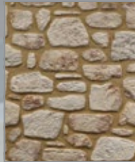
laid with mortar color "Brown Sugar"
