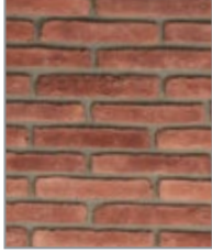
laid with mortar color "Ash Gray"
