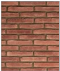
laid with mortar color "Mocca Brown"
