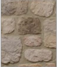
laid with mortar color "Ash Gray"
